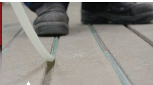
- into which the heating pipes are laid
