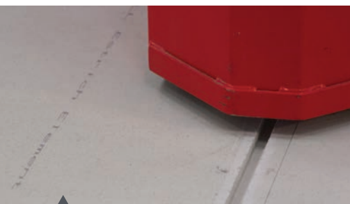
The JK Floorgrinder produces dust-free grooves in the Fermacell® floor panels -
